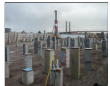
Construction work begins with 700 pre-cast concrete piles.
